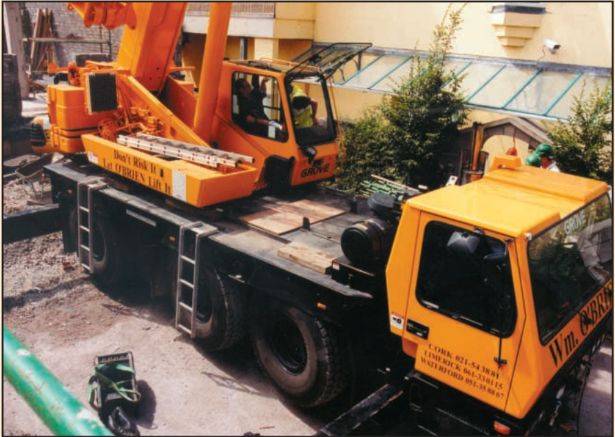
50 ton All Terrain crane at work in a confined area.
