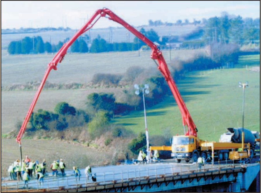
42 metre concrete pump working on a new road development.
