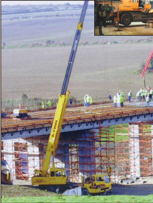
25 Ton Truck Mounted Crane.
