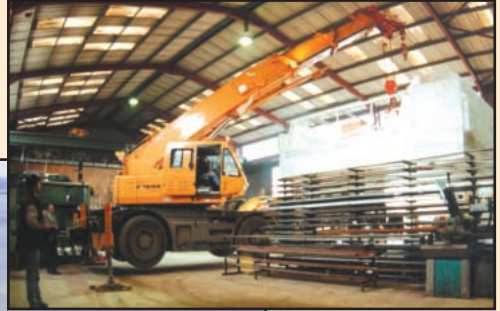
City Crane at work in a height restricted area.
